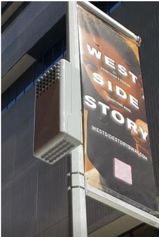
enclosure is a single-tenant solution that can hold 4G and 5G radios and supporting electronics, and all radios and components can be individually dismantled and replaced for future upgrades. Like the DoITT 4G-Only Shroud, it uses enhanced thermal management to optimize operation during New York's weather extremes.
